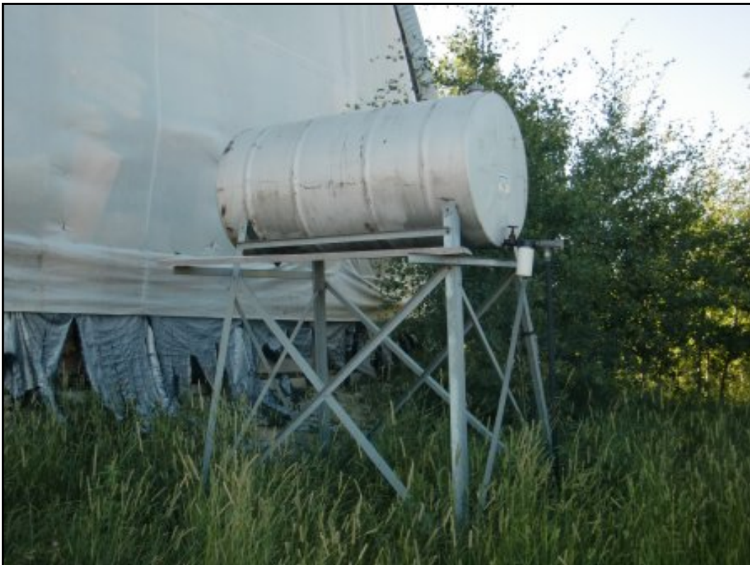
AST containing diesel fuel, located west of the hay shed.
