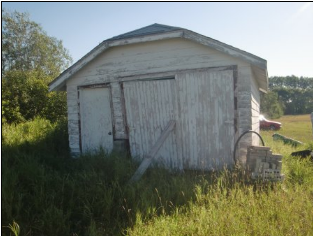
Storage shed located south of the residential property.
